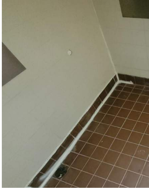
Photo 6 and 7 Cracked tiles in wall to be replaced in changing rooms
