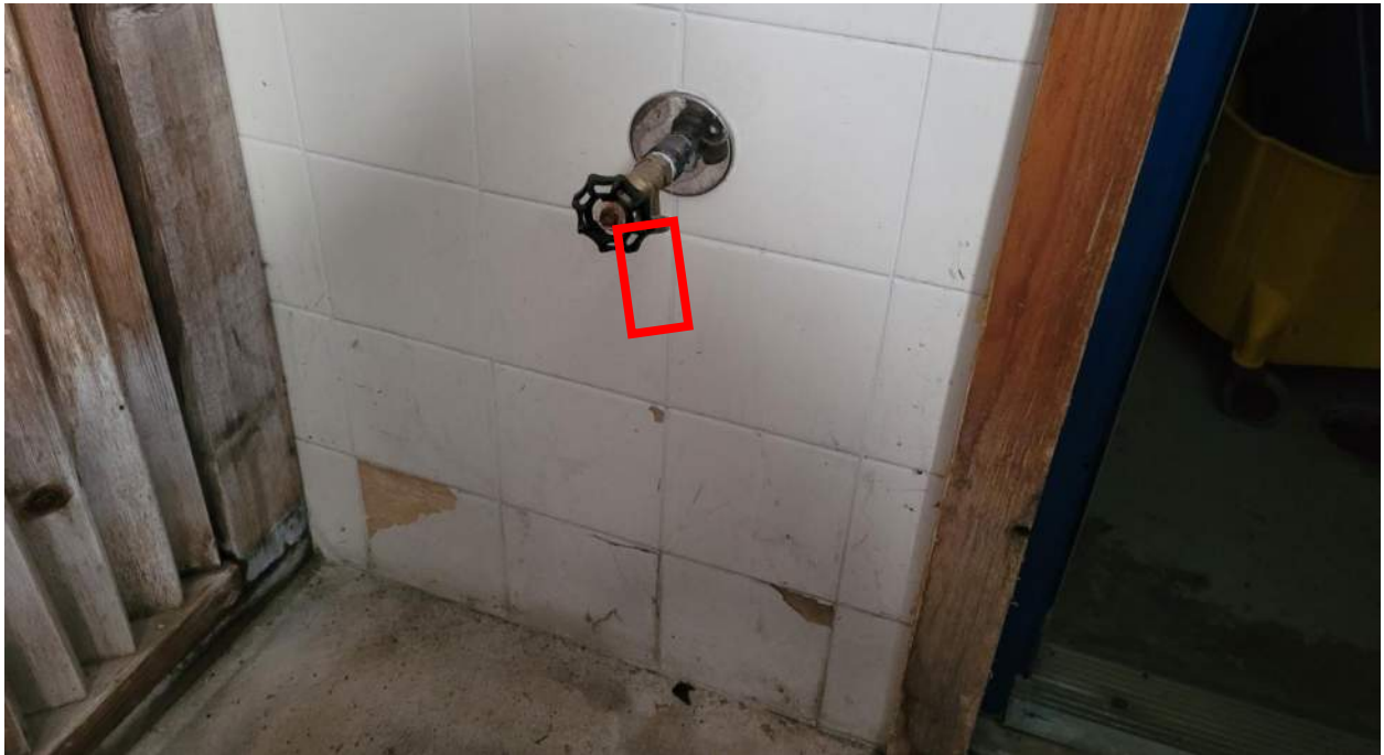
Photo 15 Install vacuum breaker on hose bibb
