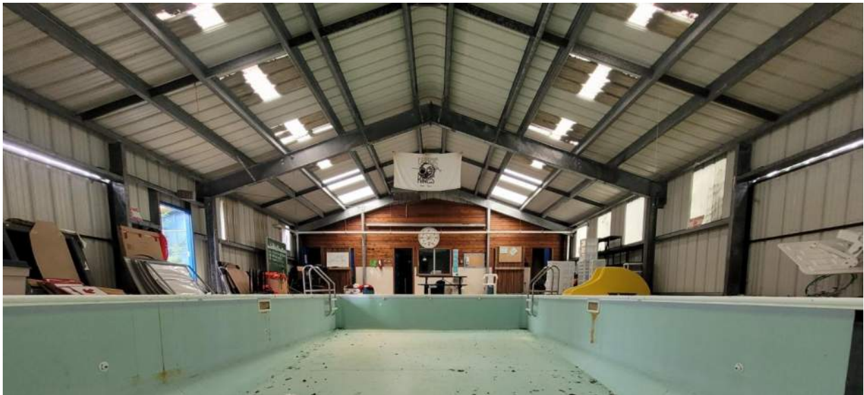
Photo 10 Remove moss from roof exterior
