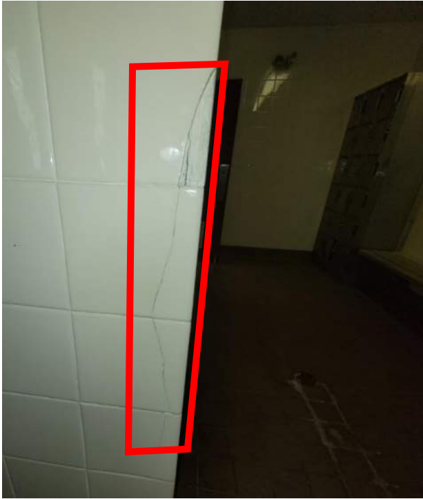
Photo 6 and 7 Cracked tiles in wall to be replaced in changing rooms
