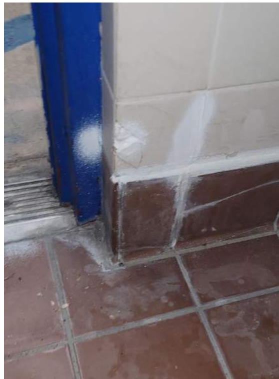
Photo 4 and 5 Cracked tiles in wall to be replaced in changing rooms
