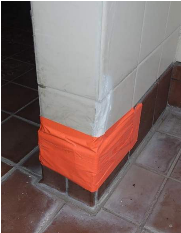
Photo 4 and 5 Cracked tiles in wall to be replaced in changing rooms
