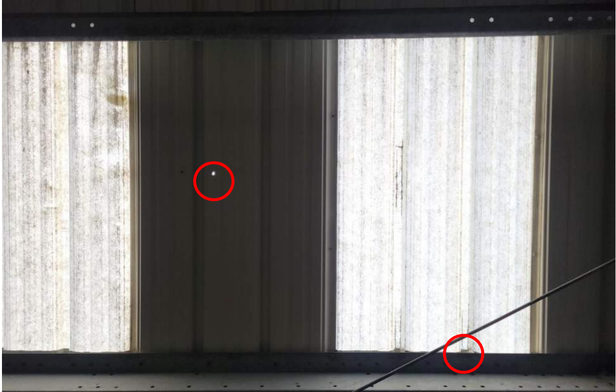
Photo 11 Repair holes in roof
