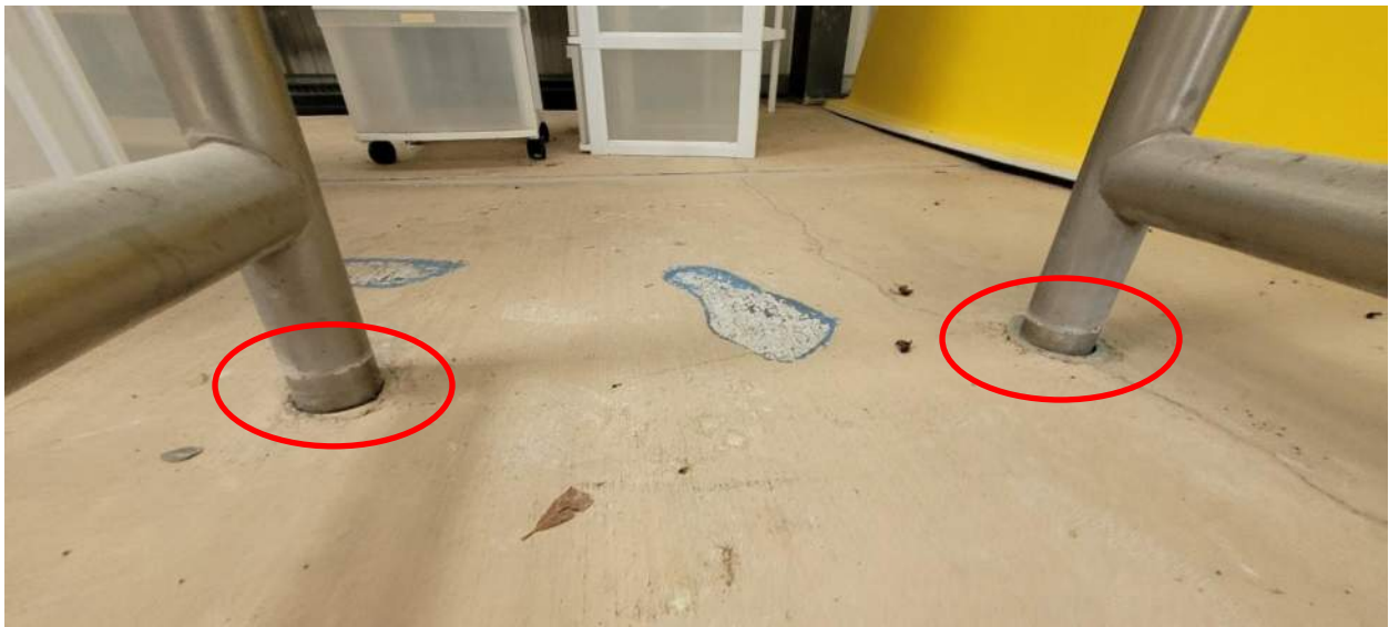
Photo 2 Escutcheon plates to be installed on each ladder
