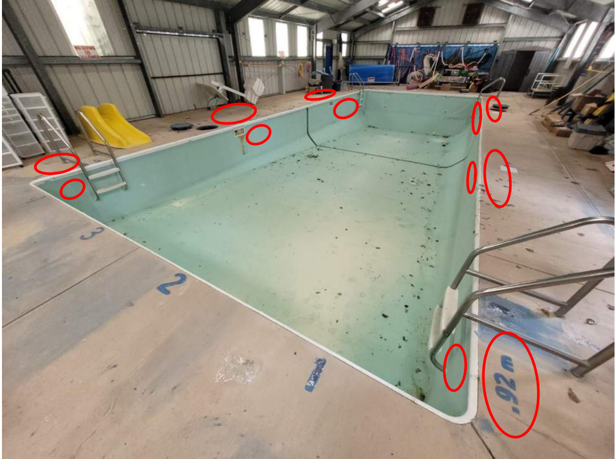
Photo 1 Depth Markings to be installed on pool deck and interior of pool above water line
