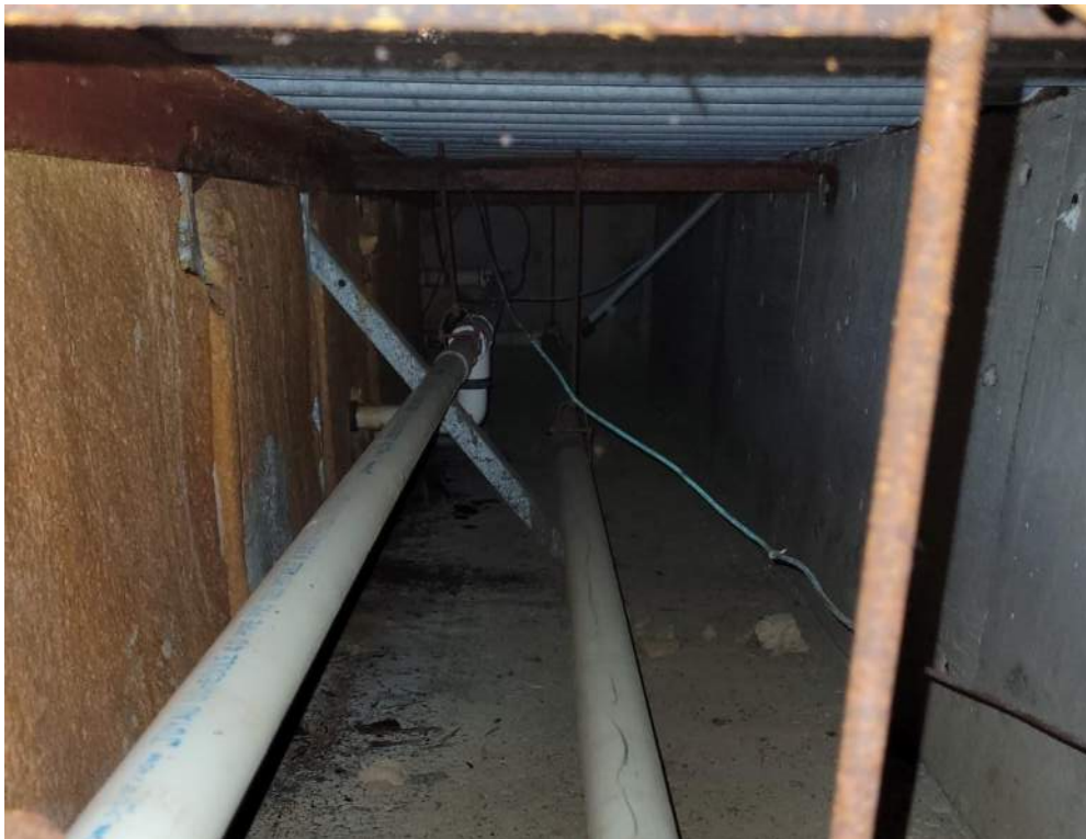
Photo 17 Install ventilation to chase around pool
