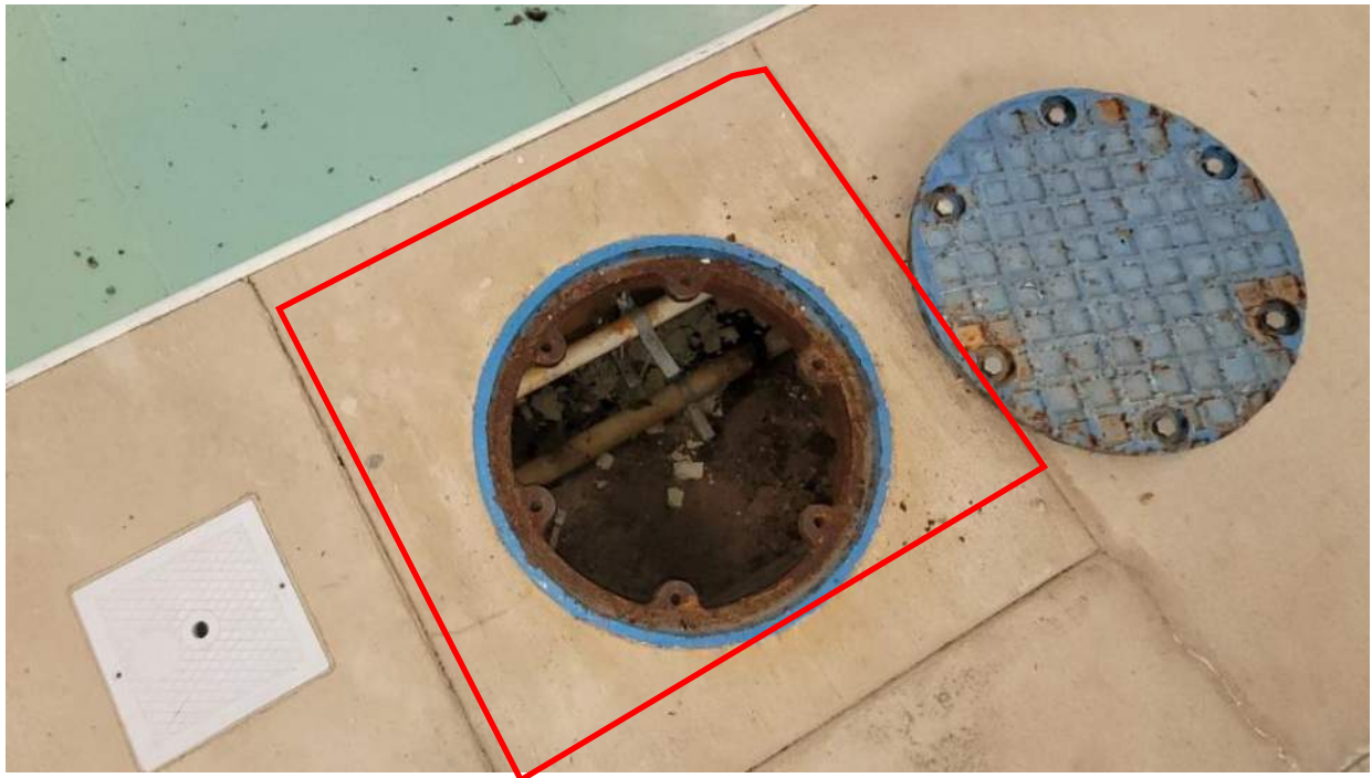
Photo 8 Remove existing access hatches and install new access hatches
