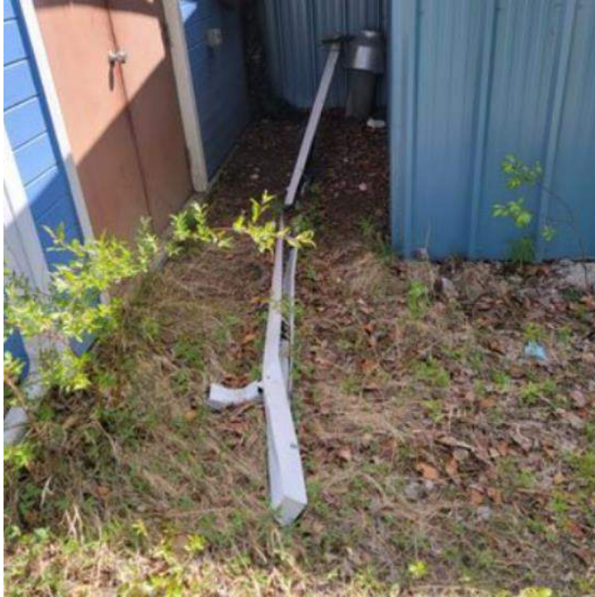
Photo 9 Replace fascia and reinstall gutter to mechanical room
