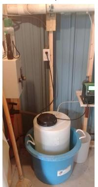
The chlorine feed system is housed in a separate room which also houses the solar heating system storage tank and circulation pump. The Grundfos chemical feed pump delivers liquid chlorine from the chemical tank and into the return piping back to the swimming pool. This pump is set to continuously dose chlorine at a set rate. The operators take regular chemical samples and readings and manually adjust the chlorine and acid as needed.
