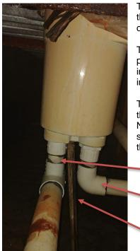
The ports in the sidewall below each skimmer are to be permanently sealed, and the skimmer equalization ports are to be plumbed to the main drain piping as close as possible to the main drains.
