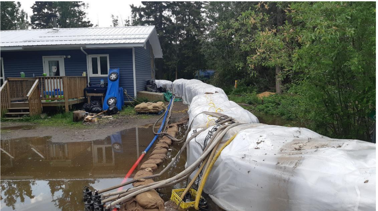
Photo 6. Residence and temporary flood protection in LSCFN lower bench, 28-JUN-2022.
