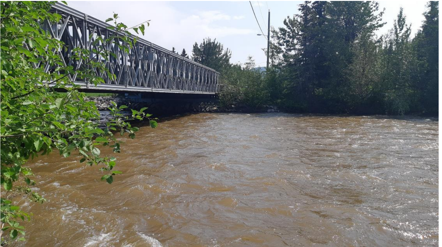
Photo 7. Nordenskiöld River bridge looking East, 28-JUN-2022.
