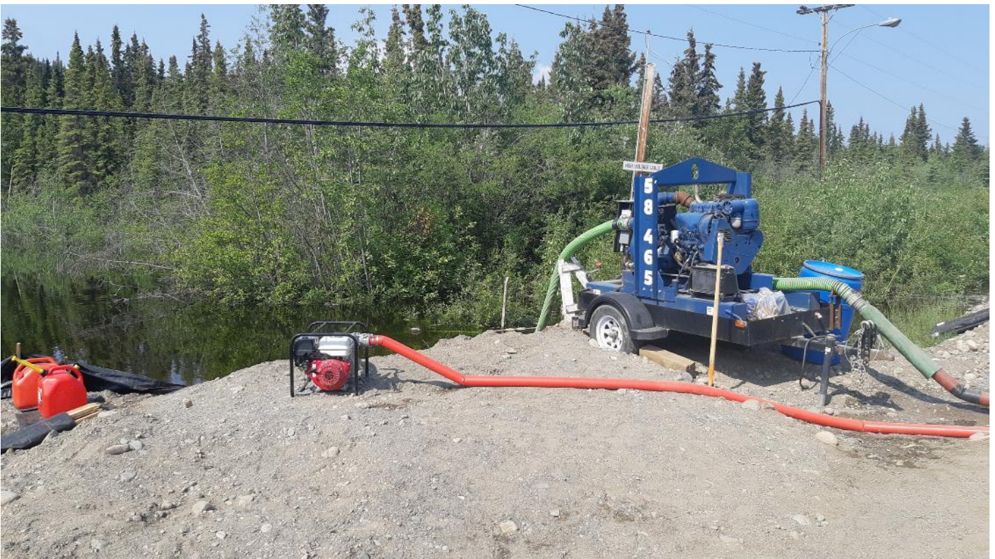
Photo 2. Diesel pump setup at location of culverts under River Drive, 28-JUN-2022.
